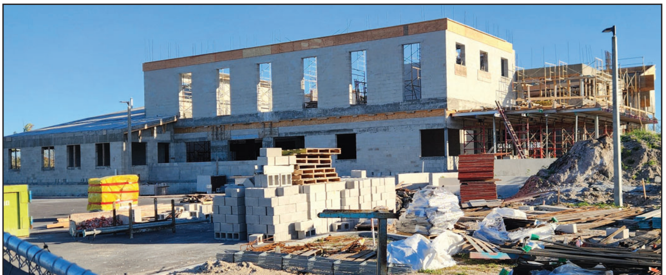
Construction of YMCA's brand new 17,000-square-foot Healthy Living Center
