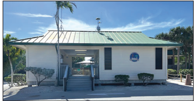
The restroom/ranger station building at Tigertail Park is slated for demolition and replacement, with new sidewalk ropes visible on the right.
