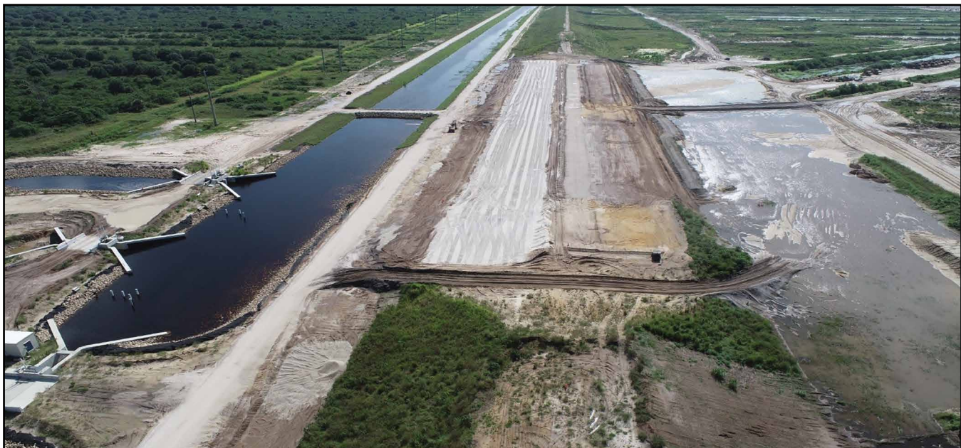
Progress on the North Embankment of the Caloosahatchee (C-43) Reservoir Project
