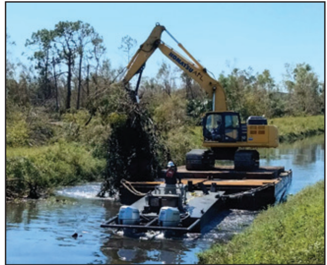
The SFWMD worked with Lee County to remove debris from the drainage system with a focus on Ten Mile Canal, Telegraph Creek, Daughtrey Creek, Orange River and Hickey Creek
