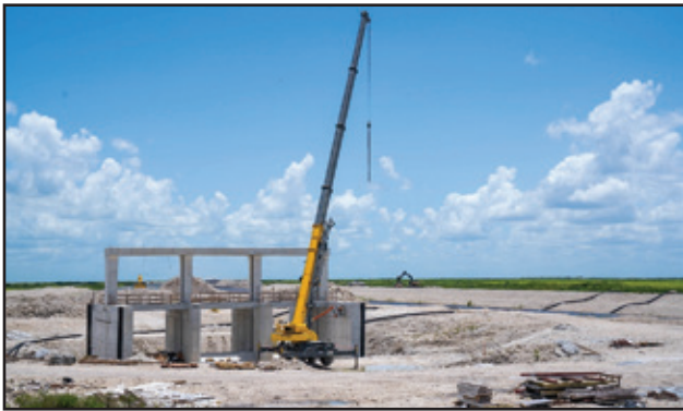
Construction at the EAA Reservoir Project Stormwater Treatment Area Water Control Structure
