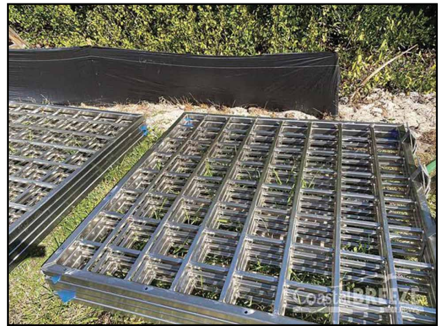
These manatee gates will be installed over the ends of the culverts to prevent manatees from being trapped
