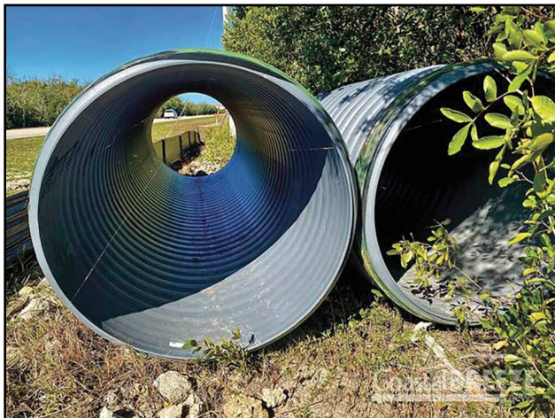
A total of four culverts will be installed under San Marco Road to provide flow to the mangroves
