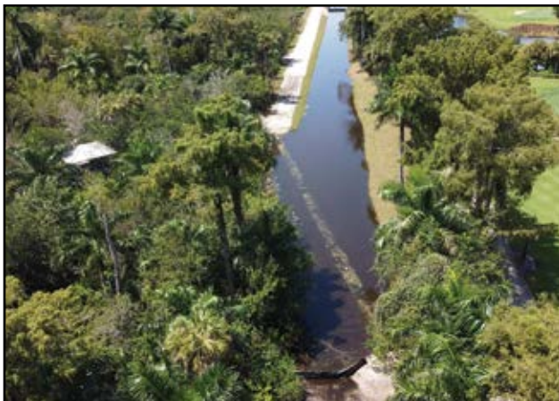
New Spreader Swale at Freedom Park in the Big Cypress Basin in Collier County
