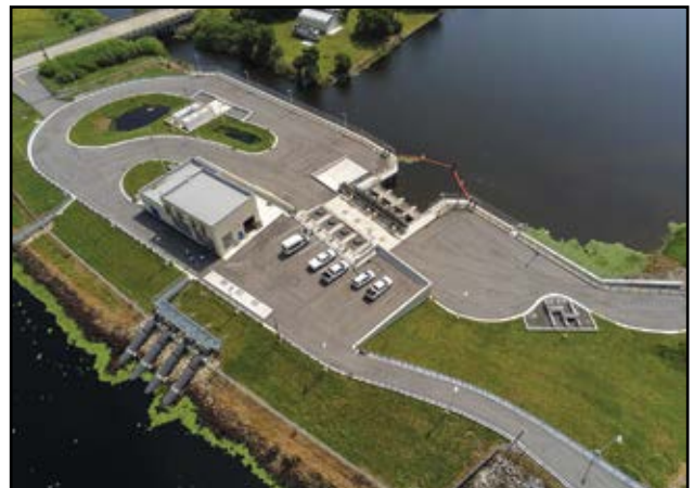
S-191A Pump Station in Okeechobee County, part of the Lakeside Ranch Stormwater Treatment Area
