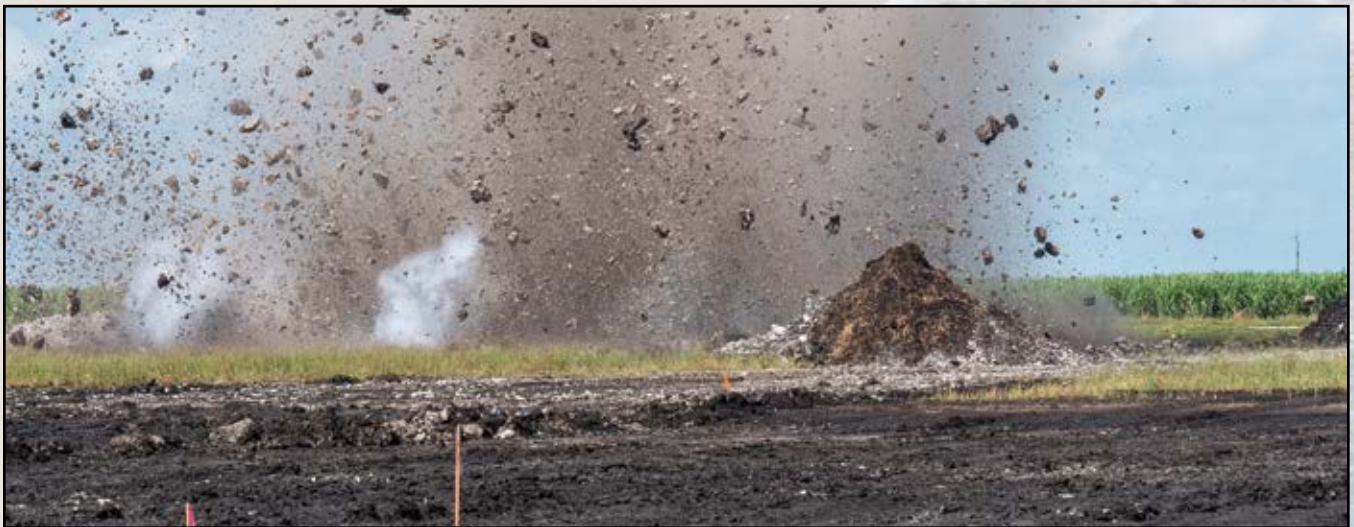
Explosives used to help excavate canals that will bring more clean water to the Everglades
