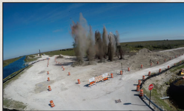
A controlled explosion to begin construction on the S-333N Structure, which will provide more water to Everglades National Park
