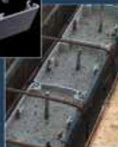
STEEL REBAR AND CONCRETE ENCASED INSIDE VINYL FORM
