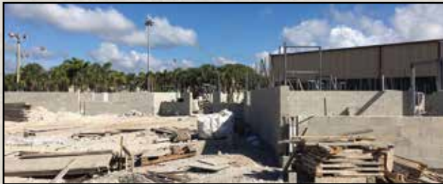
Mackle Park Community Center under construction, October 2016
