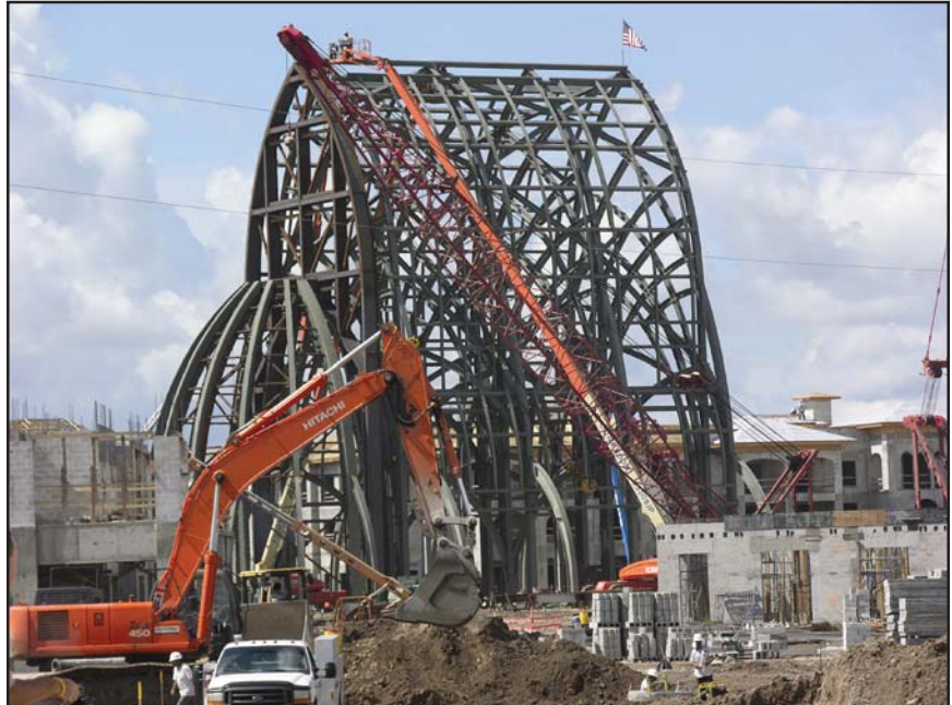
The AMU Oratory frames are raised into place as the town center of Ave Maria Florida takes shape. Photo by Ron Kerman
